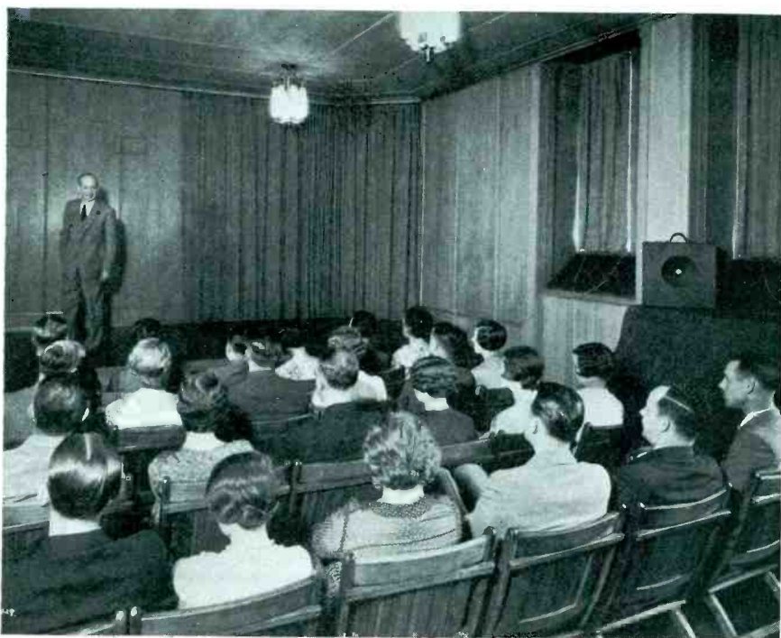
CORRECT SPEAKER POSITION —A satisfactory setup for a small installation. Notice speaker baffle placed at right angles to microphone to reduce feedback.
