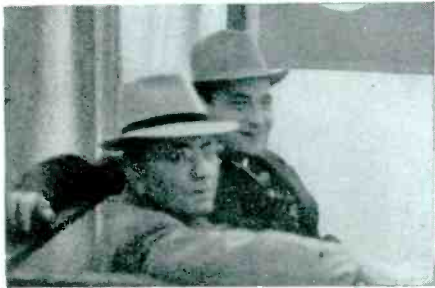
... never caught napping. KAHN of Standard Transformer (smiling, as usual) and Bill Schuler of New Orleans
